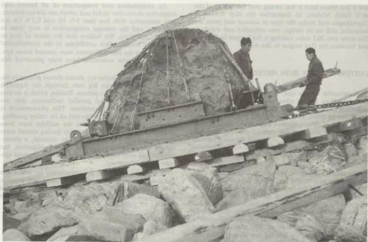
Fig. 9. The sledge of profile irons has been assembled under the meteorite, and it is now being pulled towards the beach by hand-operated winches. August 1965.
