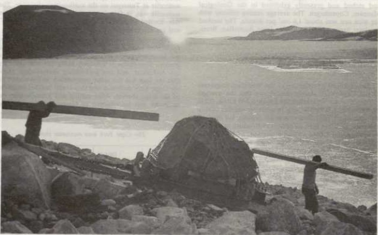
Fig. 10. A shot taken at midnight when the sun is directly north above the distant glacier. The 15 m long "rail-road" of heavy timbers was dissolved when the meteorite had passed and reconstructed in front of it saving a lot of material.
