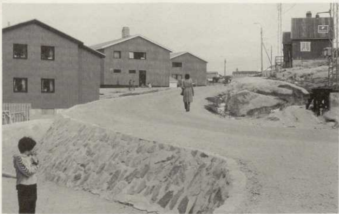
There are no roads between the individual towns. Roads in Greenland towns are to absorb internal traffic only. As part of ground care, a considerable effort is made to cover slopes and ditches with stone.
